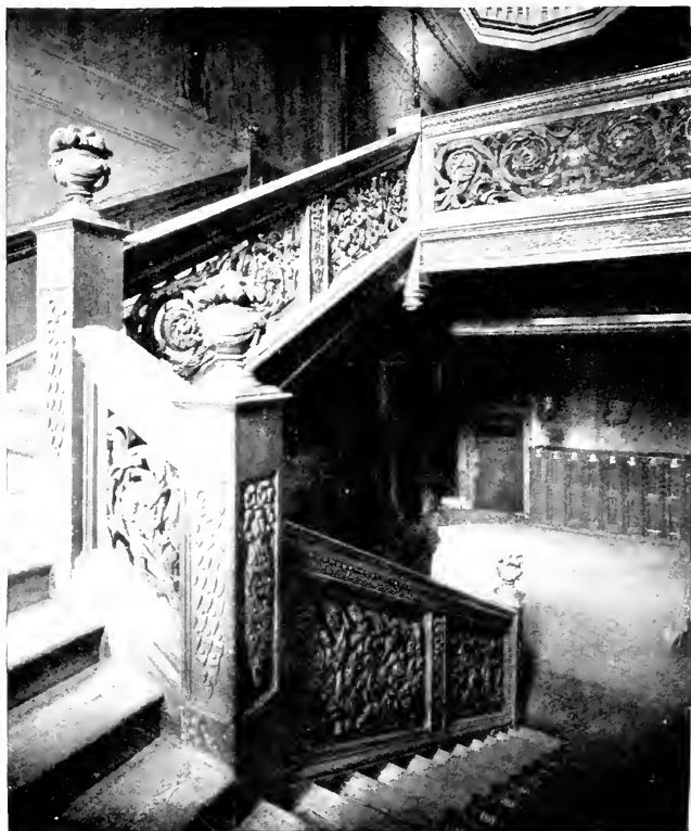
173. Staircase, Eltham Lodge.
